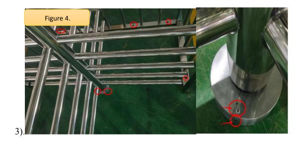
Step 4: Mark 10 expansion screw holes for guardrail installation and 4 expansion screw holes for bearing base on the floor with marker pen.
